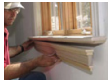
Figure 6. The 1x3 apron is wrapped with panel molding top and bottom (top right). The author glues and pins the small pieces together with a 23-gauge headless pinner (center right), then installs the apron in one piece (bottom right). The finished window (above).
