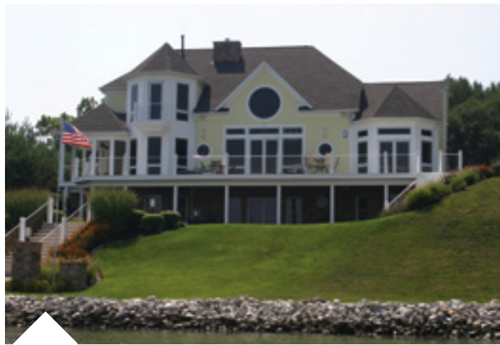
WHOLE HOUSE RENOVATION 500K - 600K SILVER MERIT Company Coastal NRM Builder Project From Uninspiring to Spectacular
