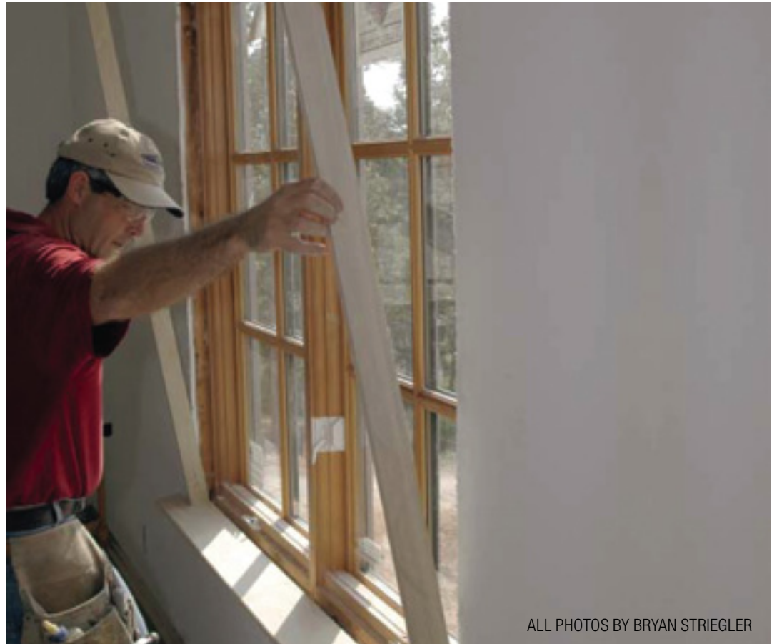
Figure 1. For the look of a traditional stool, the author uses full 1-inch-thick stock profiled with a router. He shapes the bottom edge with a cove-and-bead bit and the top edge with a 5/16-inch roundover bit. At right, the finished edge profile with the router and trimmer held in place.
