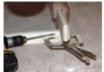
Figure 3. Pocket screws hold the jamb extensions together so they can be installed as a unit (top). On large windows the author attaches the stool with screws (bottom); on small ones he pins the stool to the side jambs from beneath.
