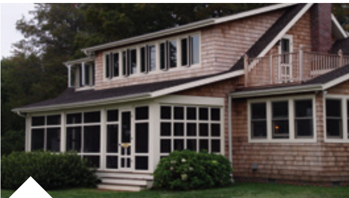
WHOLE HOUSE RENOVATION 500K - 600K AWARD OF EXCELLENCE Company JFK Construction Project Parkhurst Residence
