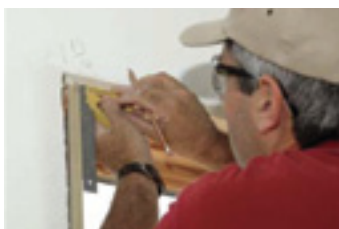
Figure 4. The author uses a level as a straightedge when shimming the stool, which results in an even reveal along the bottom edge of the window.
